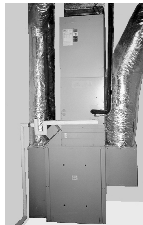
UERV Unit with Upflow Air Handler (Return Air Ducted, Outside Air and Exhaust Ducted to Outside)
